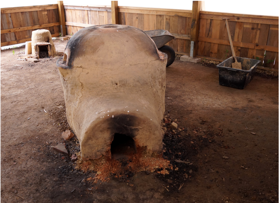
Abb. 1: Feuchtigkeitsbedingte Schäden am Ofensockel des Glas-Schmelzofens GO-Borg-1. – Damage of the glass furnace GO-Borg-1's base due to humidity.
