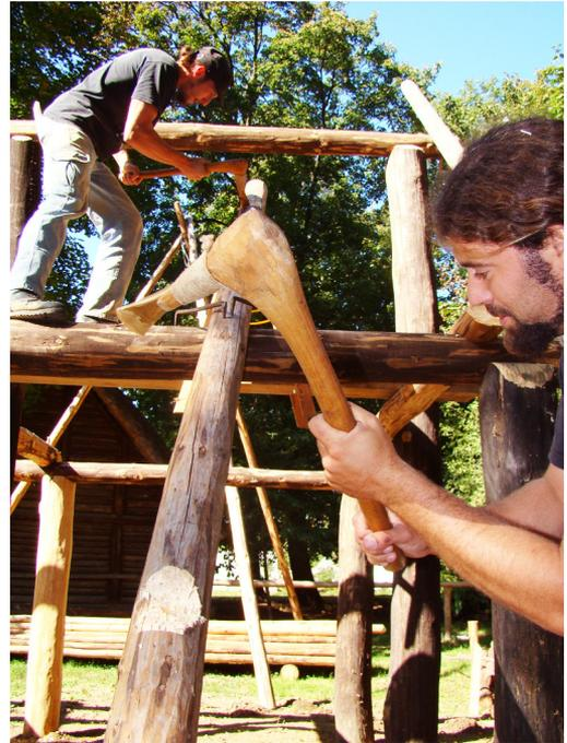
*Abb. 2: Die gewölbten Schneiden der Bronzebeile waren gut geeignet, um halbrunde Verbindungselemente an den Bauhölzern zu formen. – The curved blades of our bronze axes turned out to be very useful for carving round shaped joints on the construction woods.*
